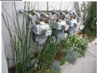
There is an automatic seismic gas shut-off for all the gas meters in the building, There is a separate shut-off for each meter. (A plumber or the gas company could determine if this is the correct size and type, and if it is correctly installed and functioning)
