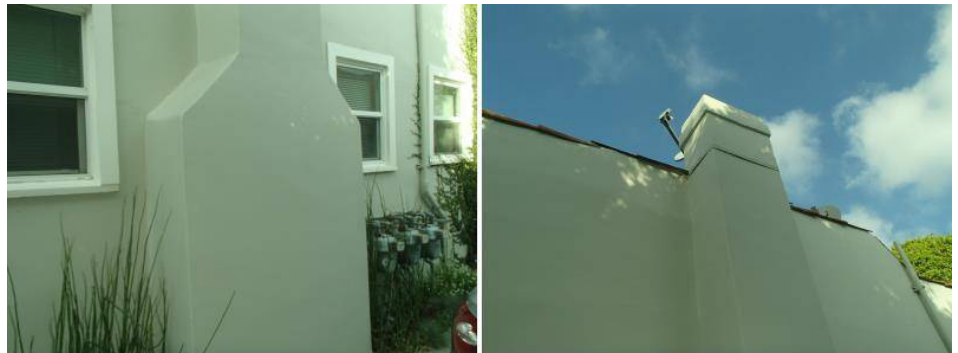
This chimney is located at the. right side.
