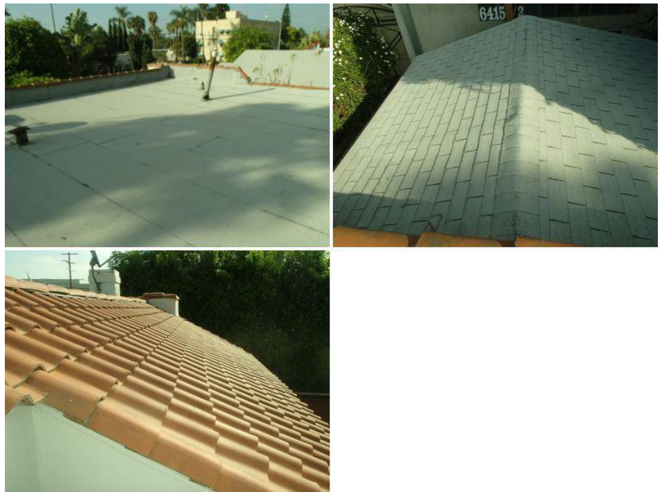
The roof is a combination of styles.
