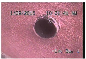
The system was accessed from a 2 inch cleanout located at the front right side of the structure off the driveway.
