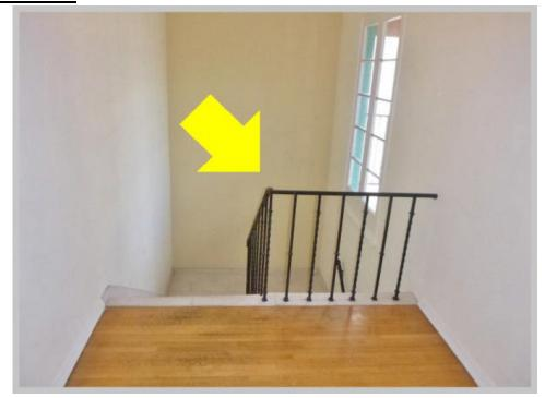
Needs Attention: The space between the rails is greater than is currently recommended for child safety. The railings should not have any space greater than four inches in any portion.
