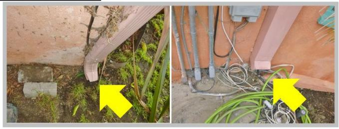
Needs Attention: The downspouts do not all route the water away from the building but instead deposit it next to the structure which can cause problems to the foundation over time.
