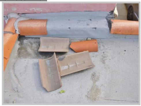
Not Acceptable: There are displaced and missing coping tiles. These can allow moisture intrusion to occur.
