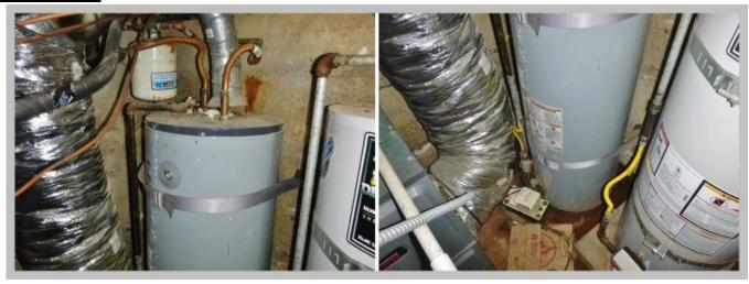
Not Acceptable: The water heater is leaking at the base.
