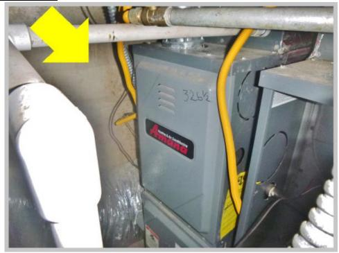
Not Acceptable: There is inadequate access space provided for service and maintenance of this unit.
