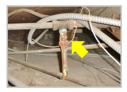
Needs Attention: The original galvanized steel pipes are rusting, corroded and are showing deterioration. These are nearing the end of the useful life and will need to be replaced in the future as these wear out. It is not possible to determine exactly when these will need to be changed out.
