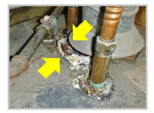
Not Acceptable: The exhaust vent line is disconnected and exhaust gases from the water heater are escaping. This is a safety hazard and needs to be repaired.
