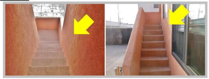
Not Acceptable: There is no handrail installed for the rear entry stairs. This is recommended for safety.
