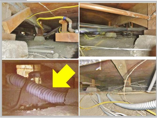
Not Acceptable: Flexible ducting is being used in the crawl space area (this duct material is only allowed to be used inside the immediate laundry area at a length of not greater than six feet). This should not pass through walls/floors or be installed in the crawl space, garage or exteriors. Smooth wall metal duct should be used.
