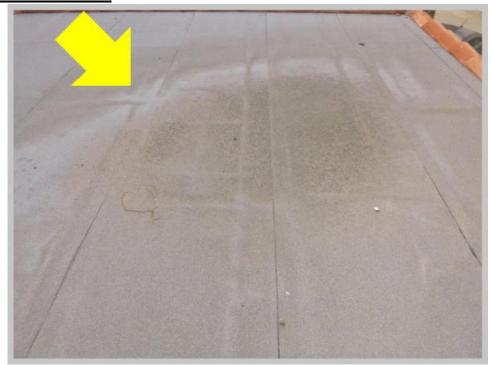
Needs Attention: On the low sloped/flat roof There are areas were the roof is poorly sloped and water collects and ponds and does not fully drain off. This can lead to premature wear and failure. A roofing specialist may be able to remedy this.
