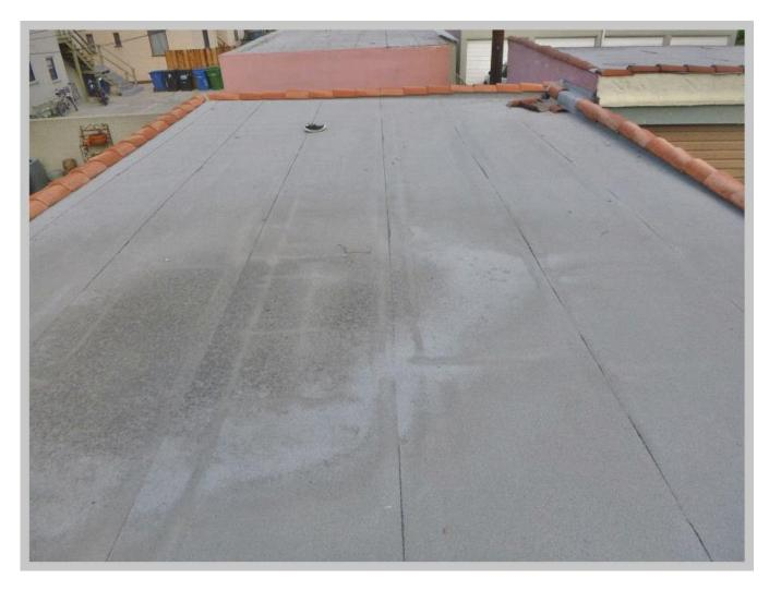
The roofing material on the low sloped roof is rolled composition roofing.
