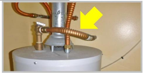
Not Acceptable: The temperature/pressure relief valve line has restrictive piping in the line. This must be approved material, so it does not malfunction.
